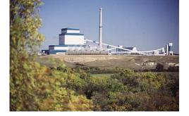
precipitator (ESP), which acts as a giant dust collector to trap over 99 per cent of the flyash before it leaves the power station's stack. Stateof-the-art computer controls ensure the plant is run as efficiently as possible
