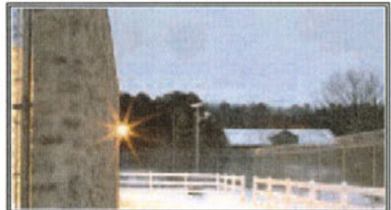
The intervention center's stone wall and rustic fence help blend the facility with the neighboring historical park. Laser intrusion technology adds security.
