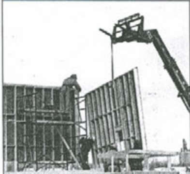
The north wall of the treatment plant is lifted into place by a crane.
