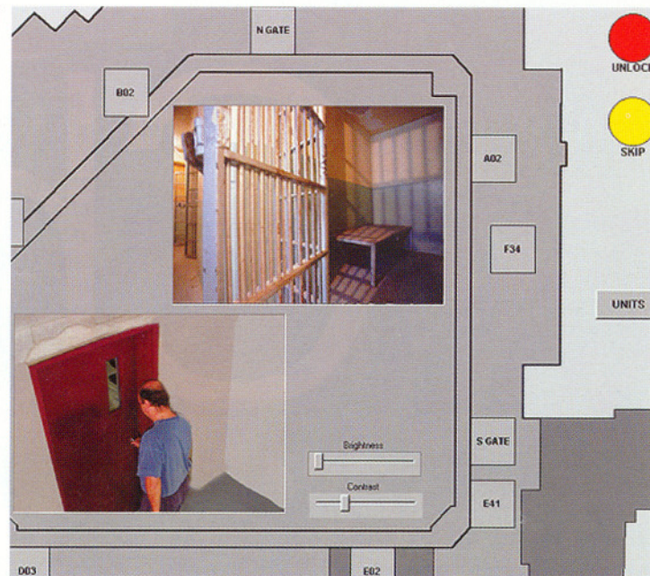
Delco Automation's touch-screen technology keeps Edmonton Institution inmates behind bars.
