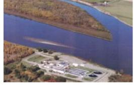
process, the wastewater passes through primary and secondary clarifiers to remove solids, two aerobic bioreactors to digest organic solids and finally through a chlorination system for disinfection prior to release to the river. In addition to the process expansion, the control system for the existing plant was incorporated into a new MCC and SCADA system.
